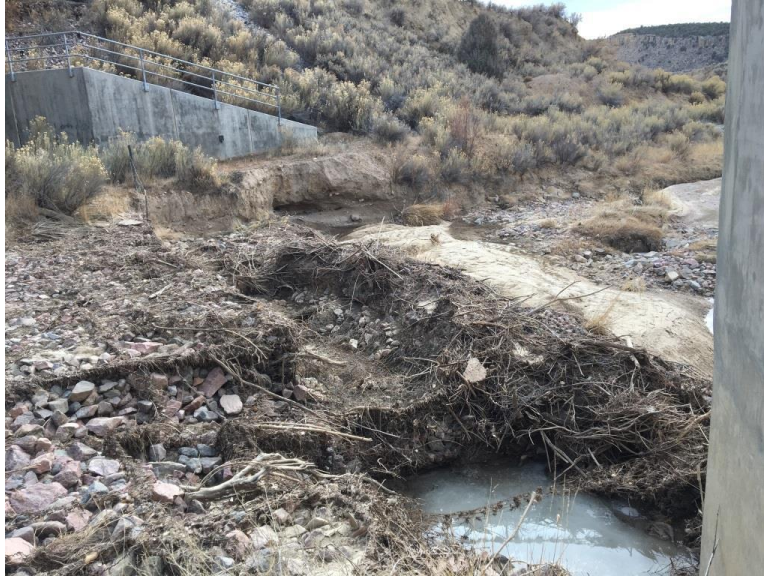
FIGURE 36 The South Rio Puerco Bridge's scour during year two of the study
