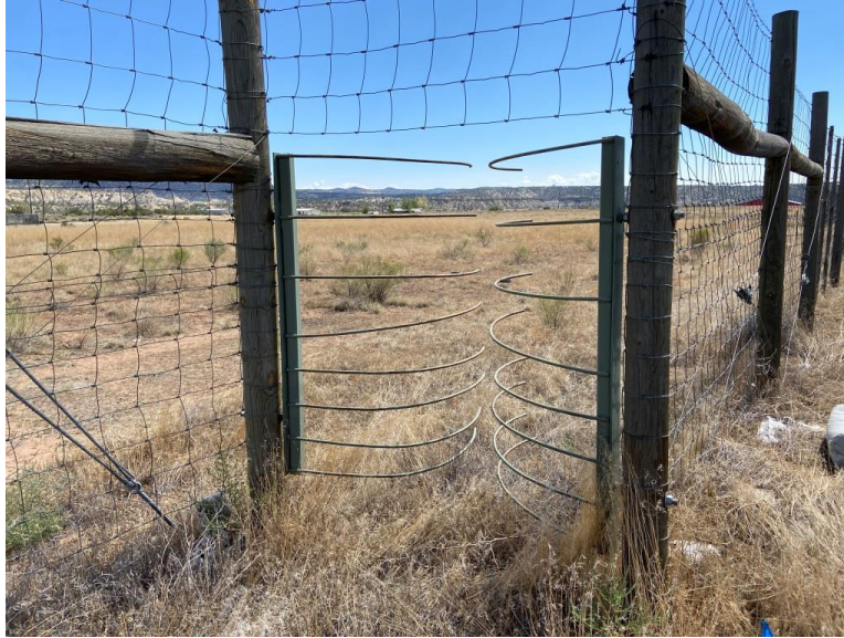
FIGURE 3 One-way gate as viewed from within the right-of-way on NM 550 near Aztec within San Juan County, New Mexico
