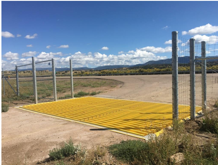
FIGURE 39 Cuba game guard on US 550 at milepost 53.5 south of Cuba within Sandoval County, New Mexico
