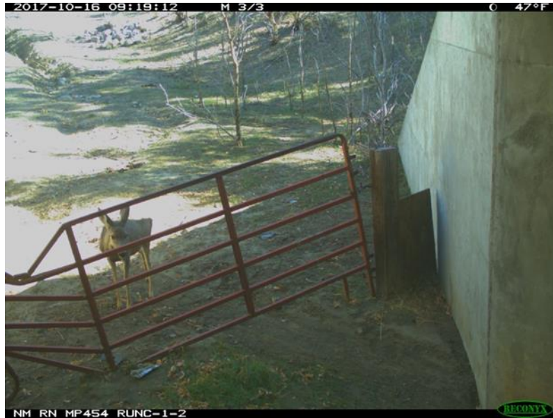
FIGURE 69 An obstruction (steel corral panel) preventing a Raton deer from using the Unnamed Concrete Box Culvert on I-25 within Colfax County, New Mexico
