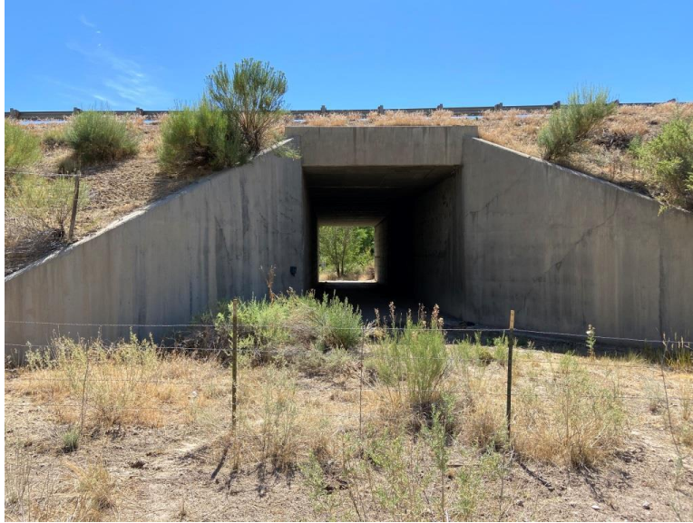
FIGURE 14 Upsized Concrete Box Culvert located at milepost 172.2 on US 550 north of Aztec within San Juan County, New Mexico
