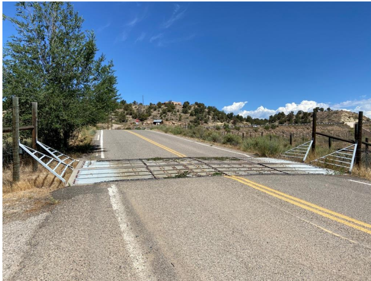
FIGURE 15 Game guard installed on US 550 on a lateral access road at milepost 170.0 north of Aztec within San Juan County, New Mexico
