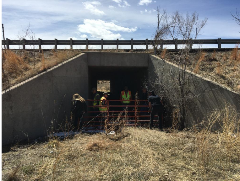
FIGURE 49 A steel corral panel obstructing a Concrete Box Culvert opening in Raton on I-25 within Colfax County, New Mexico
