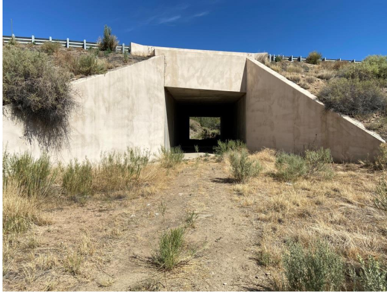
FIGURE 12 Upsized Concrete Box Culvert located at milepost 170.1 on US 550 north of Aztec within San Juan County, New Mexico
