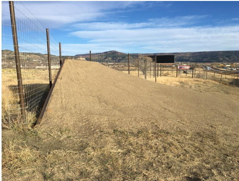
FIGURE 4 Escape ramp as viewed from within the right-of-way on I-25 at Raton within Colfax County, New Mexico
