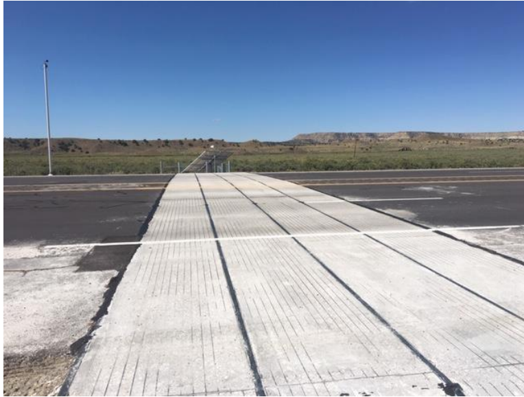
FIGURE 40 Cuba electrified barrier at game fence end on US 550 south of Cuba within Sandoval County, New Mexico
