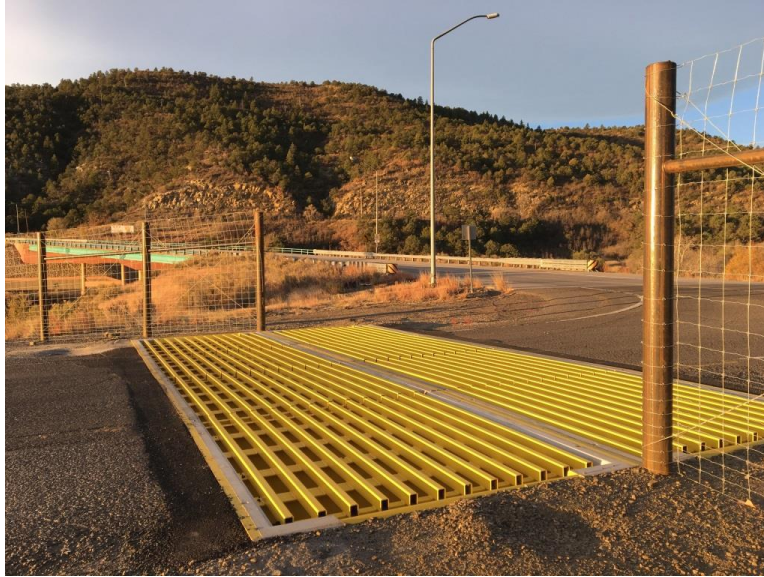
FIGURE 31 Game guard located on I-25 at the North Raton interchange within Colfax County, New Mexico
