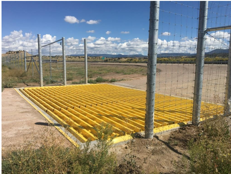
FIGURE 79 Game guard installed across a US 550 lateral access road south of Cuba within Sandoval County, New Mexico
