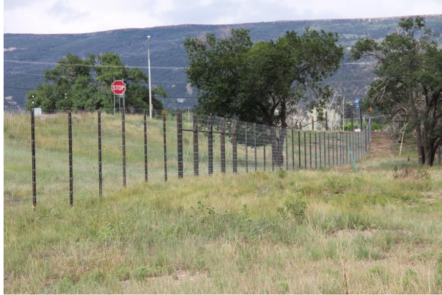
FIGURE 29 Raton game fencing on I-25 within Colfax County, New Mexico
