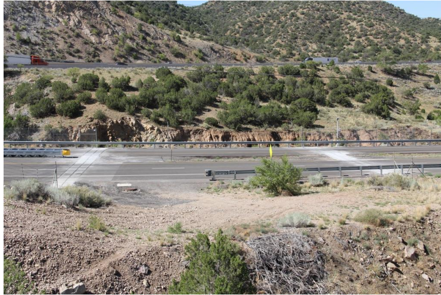
FIGURE 9 At-grade wildlife crosswalk with electrified barriers (light colored concrete) located on NM 333 at milepost 4.2 within Bernalillo County, New Mexico
