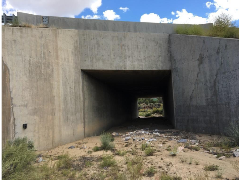
FIGURE 7 Upsized Concrete Box Culvert located on US 550 at milepost 171 north of Aztec within San Juan County, New Mexico
