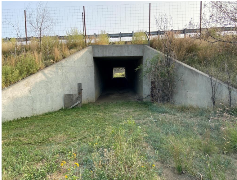
FIGURE 28 The Unnamed Concrete Box Culvert on I-25 at milepost 454.2 within Colfax County, New Mexico
