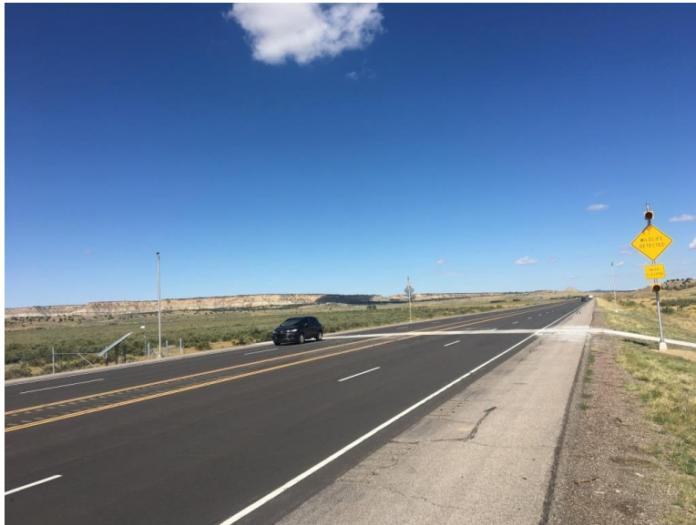
FIGURE 41 Cuba Animal Detection System on US 550 south of Cuba within Sandoval County, New Mexico
