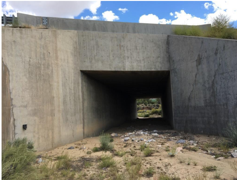
FIGURE 13 Upsized Concrete Box Culvert located at milepost 171.1 on US 550 north of Aztec within San Juan County, New Mexico
