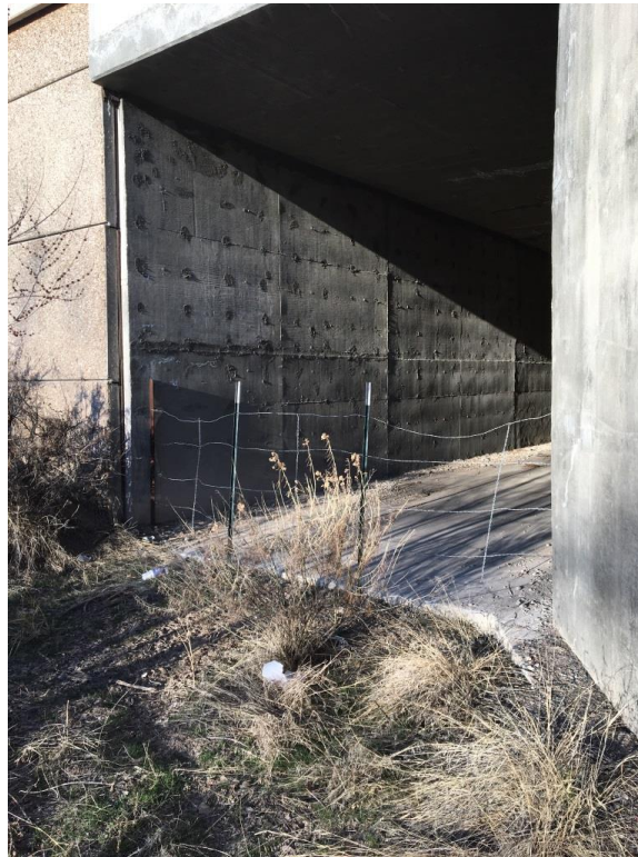
FIGURE 50 A barbed wire fence obstructing a Concrete Box Culvert opening north of Aztec on US 550 within San Juan County, New Mexico
