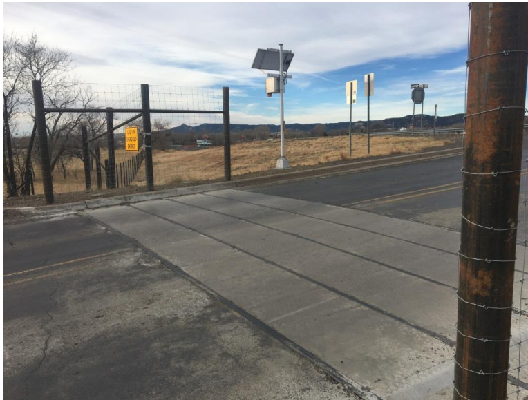
FIGURE 32 Electrified barrier on the East Cook Avenue - I-25 traffic interchange in Raton within Colfax County, New Mexico
