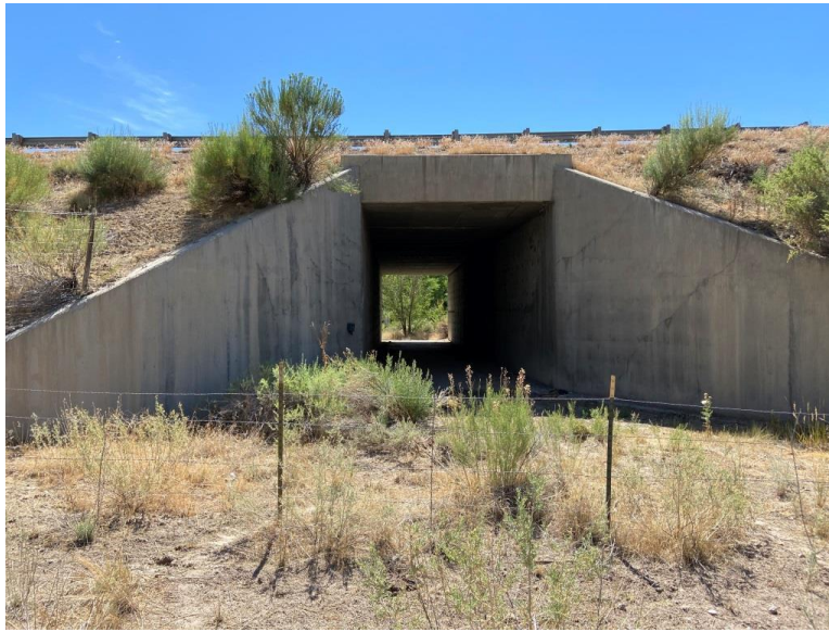
FIGURE 82 A wildlife friendly fence placed on the right-of-way boundary near an upsized CBC north of Aztec on US 550 within San Juan County, New Mexico
