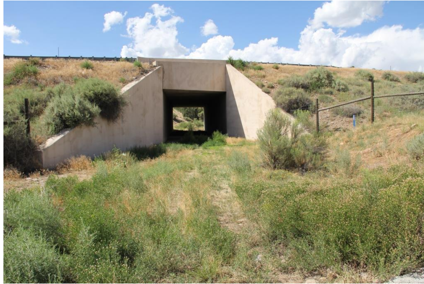
FIGURE 77 The upsized Concrete Box Culvert (16-ft tall x 20-ft wide x 120-ft long) located on US 550 north of Aztec within San Juan County, New Mexico is adequate for mule deer passage
