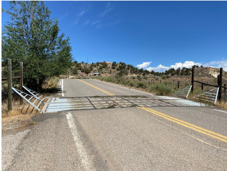
FIGURE 47 Monitored game guard north of Aztec on US 550 within San Juan County, New Mexico
