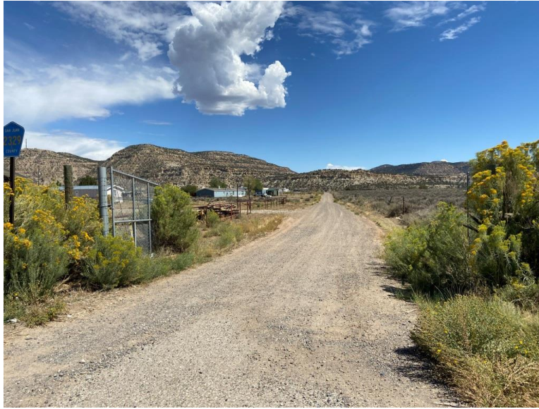
FIGURE 44 Vegetation precluded an Aztec game fence gate from closing north of Aztec on US 550 within San Juan County, New Mexico
