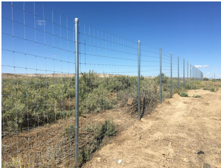
FIGURE 37 Cuba game fencing on US 550 south of Cuba within Sandoval County, New Mexico
