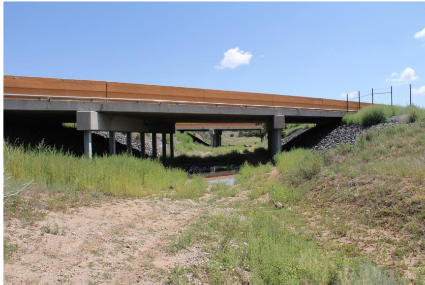
FIGURE 8 Game fencing tied to existing bridge located on I-40 at milepost 184.7 within Santa Fe County, New Mexico
