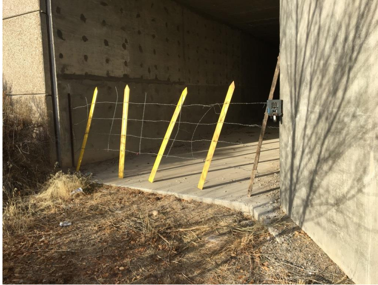
FIGURE 80 A barbed wire fence obstructing a CBC opening north of Aztec on US 550 within San Juan County, New Mexico
